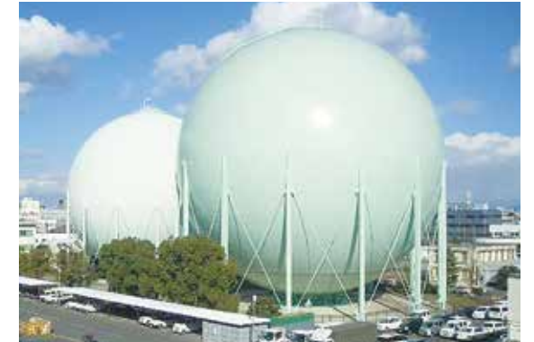
▲ A gas holder used for balancing supply and demand (Photo courtesy of TOHO GAS NETWORK Co., Ltd.)
