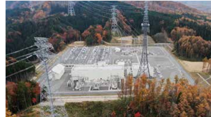
▲ The Hida Converter Station, which converts electric power frequency (Photo courtesy of Chubu Electric Power Grid Co.,Inc.)
