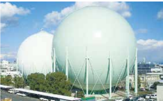
▲Gas holders for adjusting supply and demand (Photo courtesy of the Toho Gas Network Co., Ltd.)
