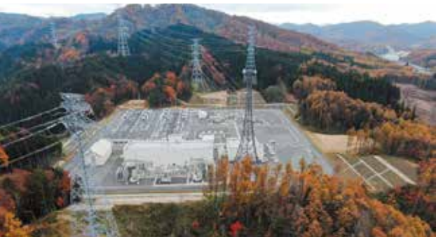
▲The Hida Converter Station that can convert frequencies (Photo courtesy of the Chubu Electric Power Grid)
